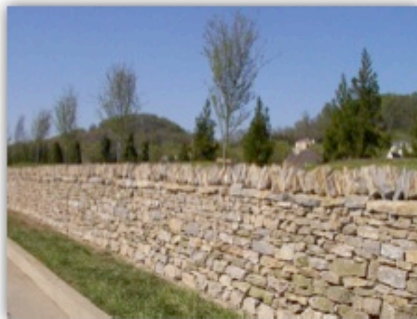
Hillsboro Road Stone Wall
